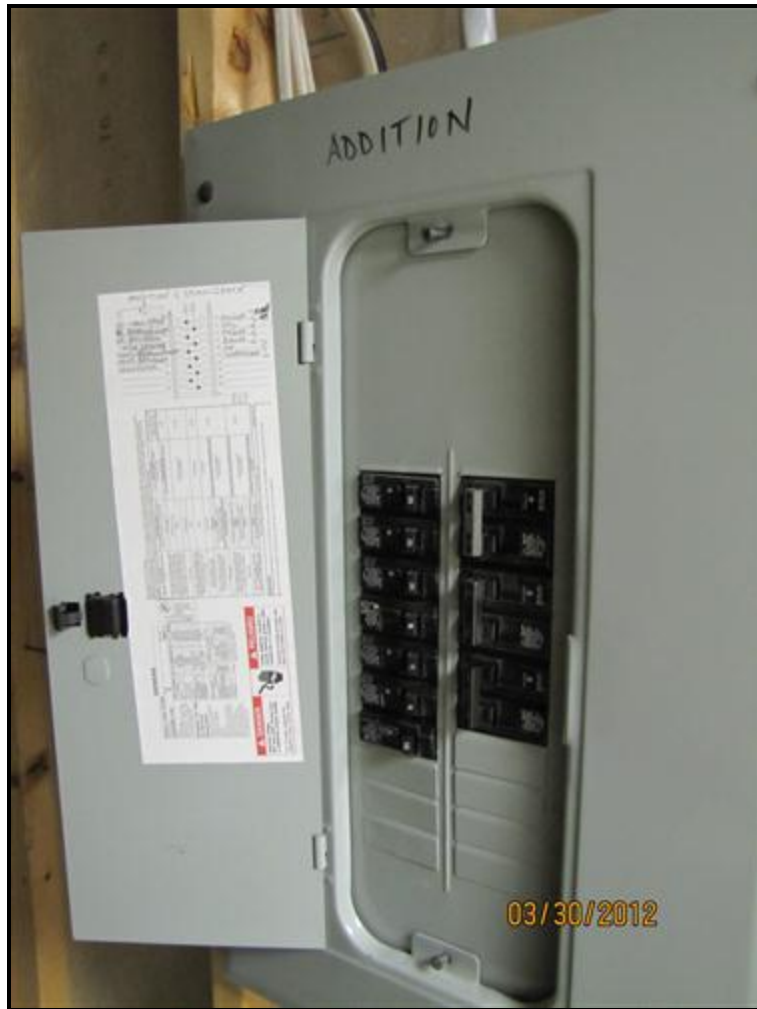
7.9 Picture 3 Secondary Panel for Addition
