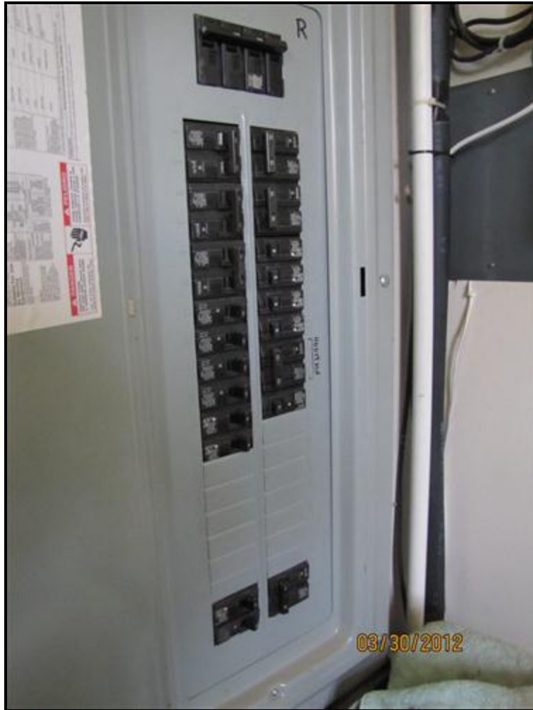
7.9 Picture 1 Main Panel
