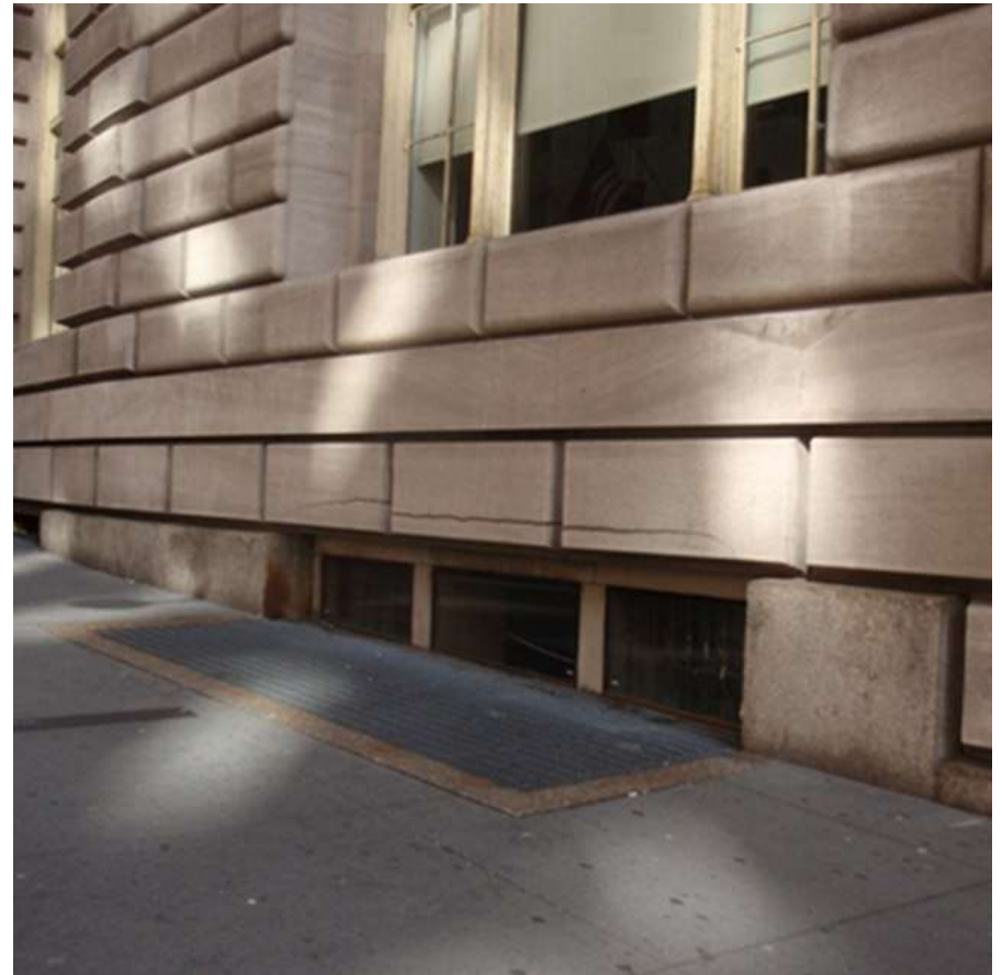
Horizontal Crack
