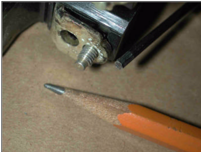
FIGURE 7 - ONE LOAD-SIDE CONTACT AND ITS 8-32 CLAMPING SCREW, ON THE FPE 100-AMP MAIN BREAKER OF FIG. 6. THE SCREW-HEAD TAKES A 3/32" ALLEN WRENCH, WHICH IS ONLY SLIGHTLY LARGER THAN THE LEAD OF THE #2 PENCIL.
