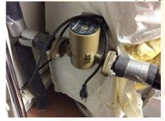
**304:** - The hot water system is equipped with a pump intended to circulate the hot water through a loop so that hot water is never far from any fixture. The system was not functioning at the time of this inspection.
