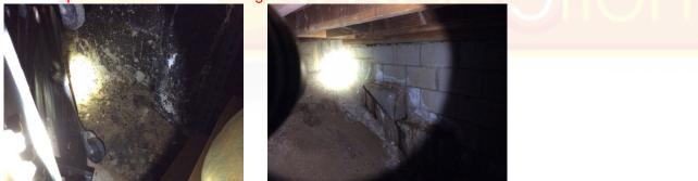
**98:** - The soil at some areas was damp at the time of this inspection. With the lack of recent rainfall, this condition is most likely a result of over-watering of the landscaping.
