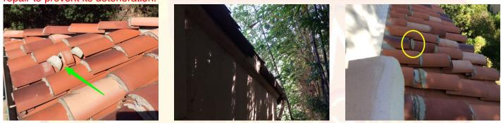
27: - There are a significant number of loose and missing tiles on the ridge and throughout the field.
