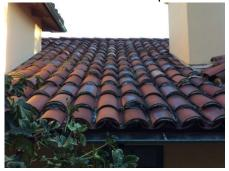
**26:** There are many individual cracked, chipped and displaced tiles along in the field. Several missing tiles is also observed. The number of affected tiles is small, but felt underlayment is exposed and we recommend repair to prevent its deterioration.
