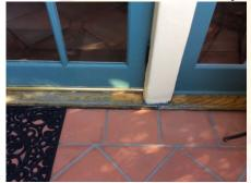
**68:** - The outward opening doors are non-preferred with regard to security and water tightness. Installation locking hinges at the doors should be considered.
