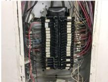
**316:** - The circuits in the subpanel are labeled. We did not verify the accuracy of the labeling, but it appears to be typical. When the opportunity arises, we suggest checking the labeling by actually operating the breakers.
