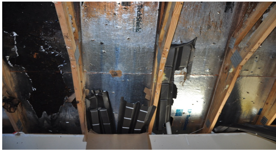
Photo 4 – Typical Evidence Observed in a Radiant Barrier Sheathing Fire Investigation Note That There are Actually Three “Ignition” Points in This Photo
