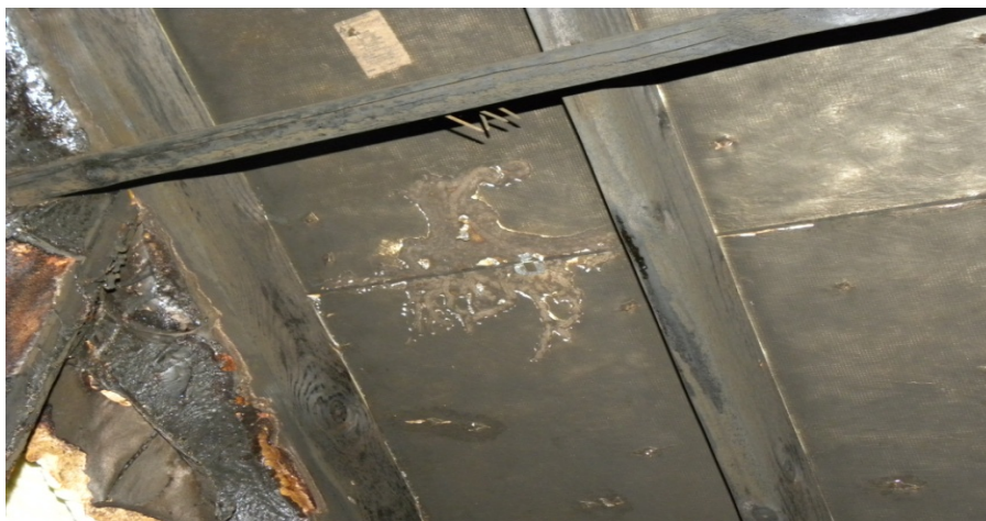
Photo 5 – A Large Arc Flash Pattern Where Extremely High Temperatures Were Generated
