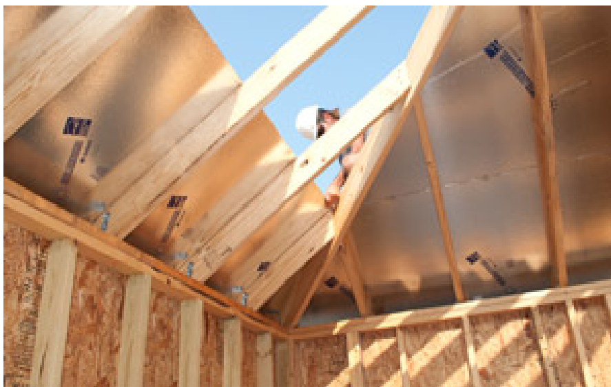
Figure 1 – Typical Radiant Barrier Sheathing Installation as the Roof Deck ( www.norbord.com )
