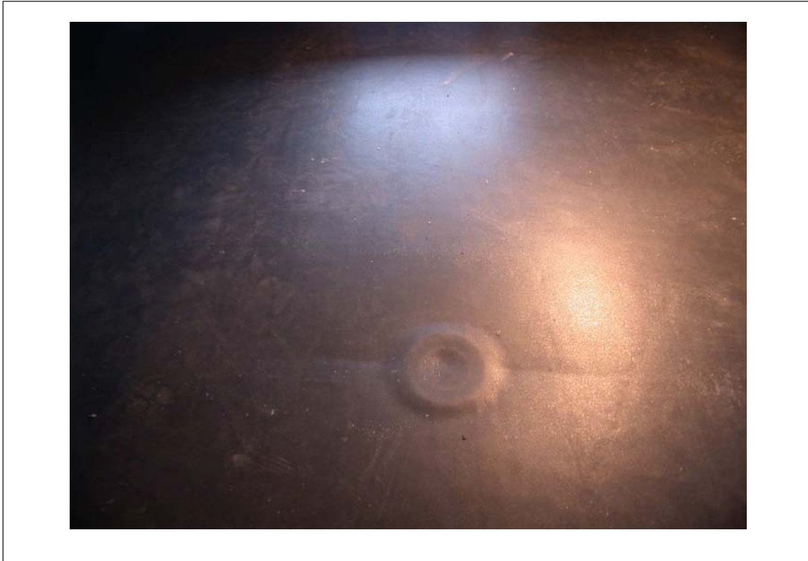
Fig. 2. Crease in single-ply roof cover while subjected to uplift pressure
