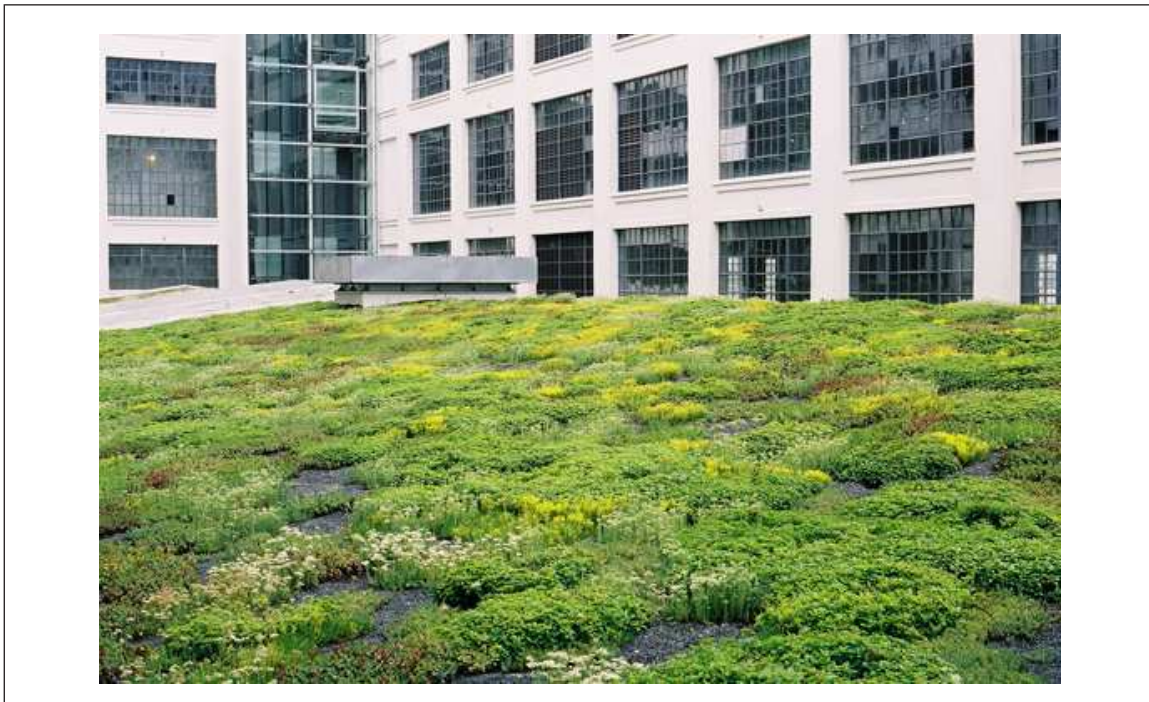
Fig. 9. Extensive green roof 2 years after installation; Montgomery Park Business Center, Baltimore, Maryland, USA (Courtesy of Katrin Scholz-Barth)
