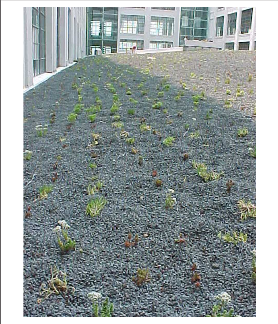
Fig. 7. Extensive green roof at time of installation; Montgomery Park Business Center, Baltimore, Maryland, USA (Courtesy of Katrin Scholz-Barth).
