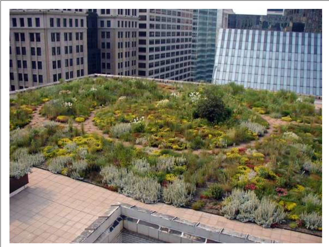
Fig. 4. Extensive green roof, Chicago City Hall, Chicago, Illinois, USA (C 2005, Roofscapes, Inc., used by permission; all rights reserved)
