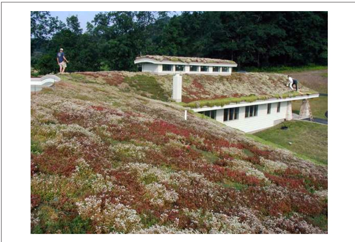
Fig. 6. Extensive green roof Life Expression Wellness Center, Sugar Load, Pennsylvania, USA (C 2005, Roofscapes, Inc., used by permission; all rights reserved)
