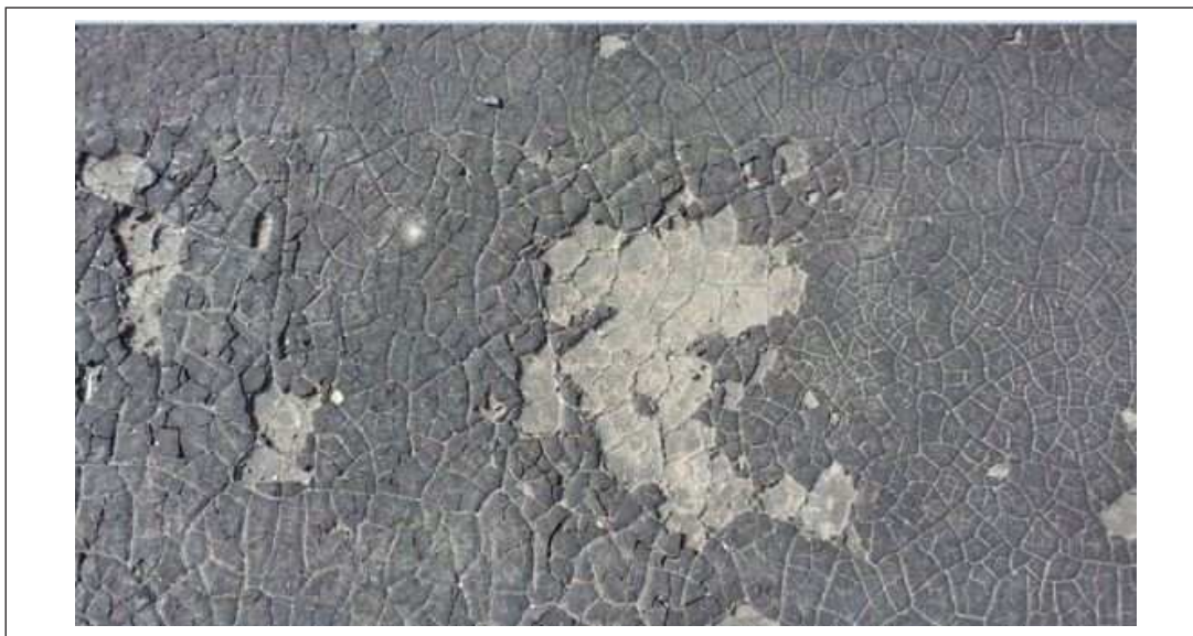
Fig. 2.3.1.2-2. Close-up of hail damage to severely 'alligatored' roof (built-up roof)
