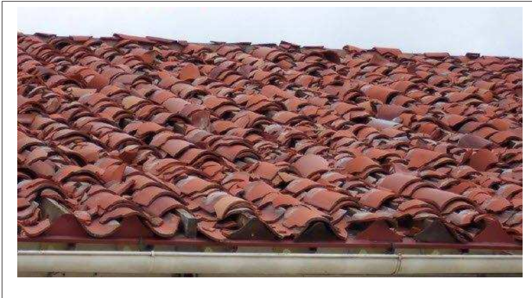
Fig. 3.4-2. Hail damage to clay roof tiles
