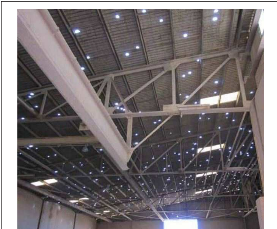
Fig. 3.4-1. Hail damage to asbestos cement roof
