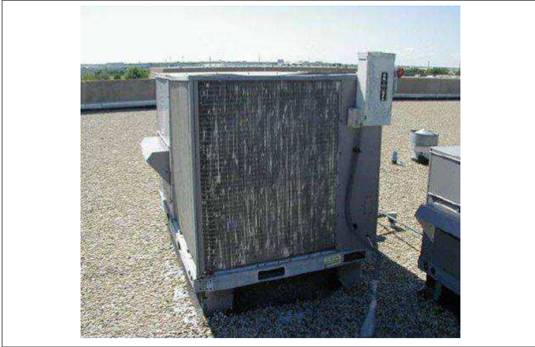
Fig. 3.1.1-1. Hail damaged HVAC unit
