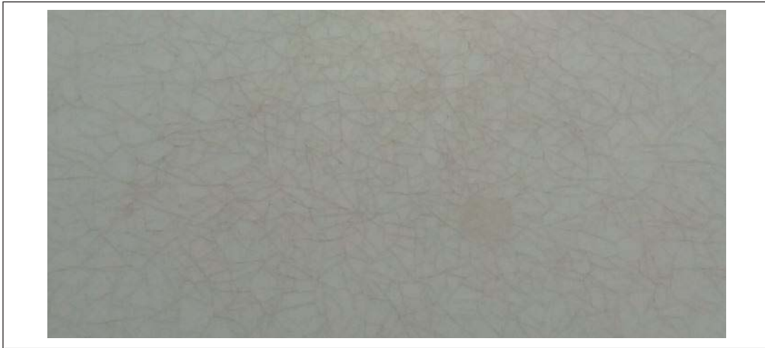
Fig. 3.1.4-3. Close up of embrittled acrylic skylight in Fig. 3.1.4-2
