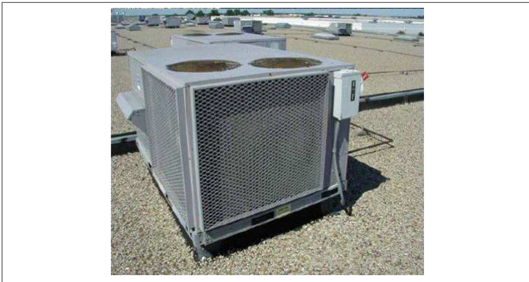
Fig. 3.1.1-2. HVAC unit with hail guard over condenser cooling fins at same location as hail damaged unit in Figure 3.1.1-1
