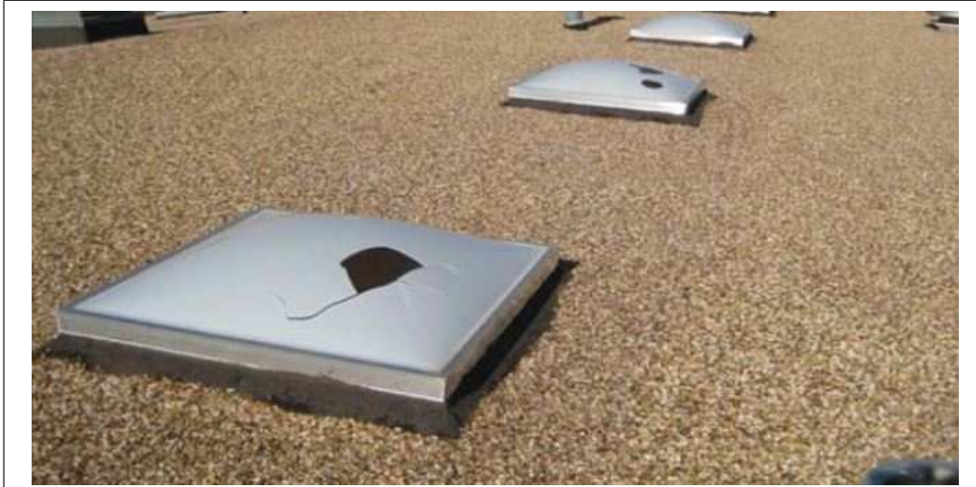
Fig. 3.1.4-1. Holes in acrylic skylights caused by hail
