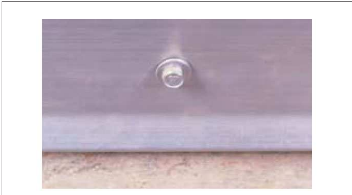
Fig. 2. Existing perimeter flashing secured at its lower edge
