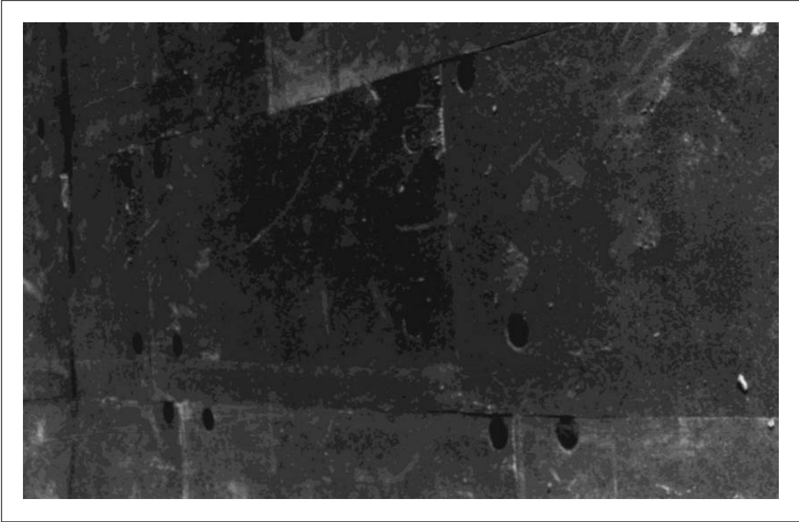
Fig. 11. Fasteners driven too close to insulation board edge
