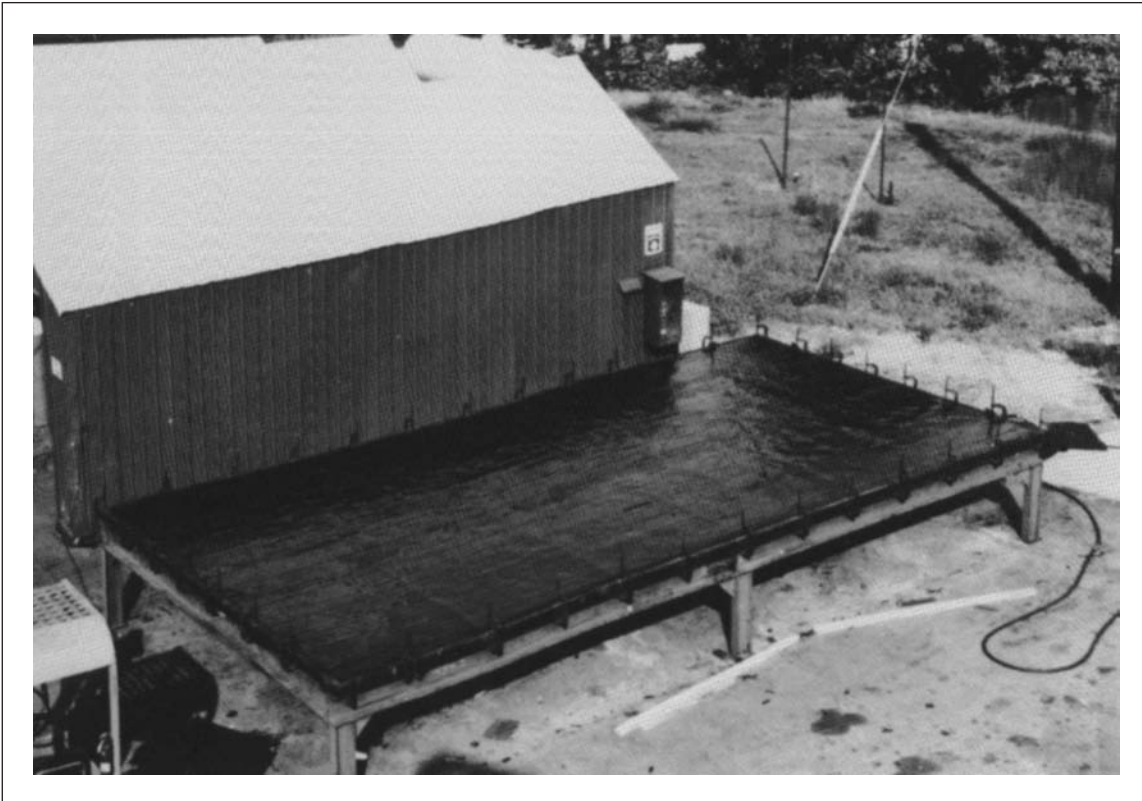
Fig. 3. Uplift pressure test samples and equipment 12.5 × 24.25-ft (3.8 × 7.4 m) test apparatus
