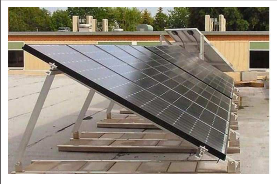
Fig. 8. Solar panels with steeper slopes or lacking wind deflectors will experience greater wind effects
