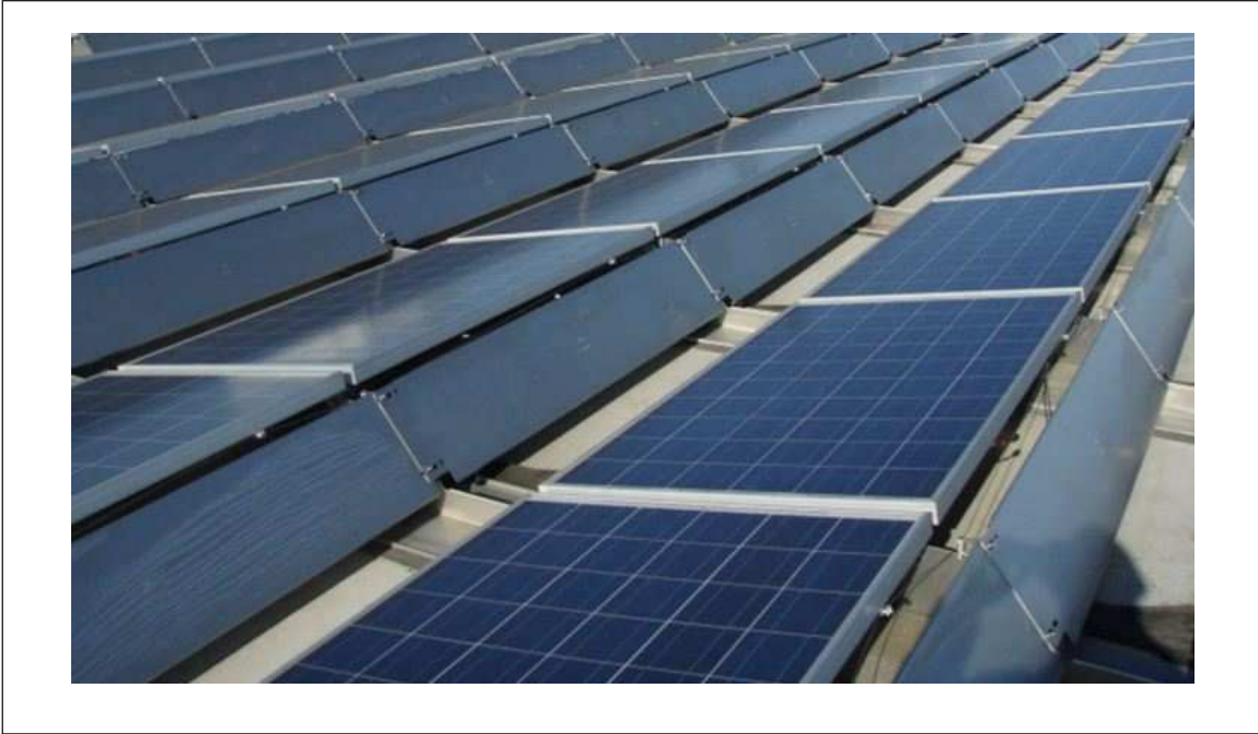
Fig. 1. Wind deflectors provided on the high sides of panels in each row (closed array)
