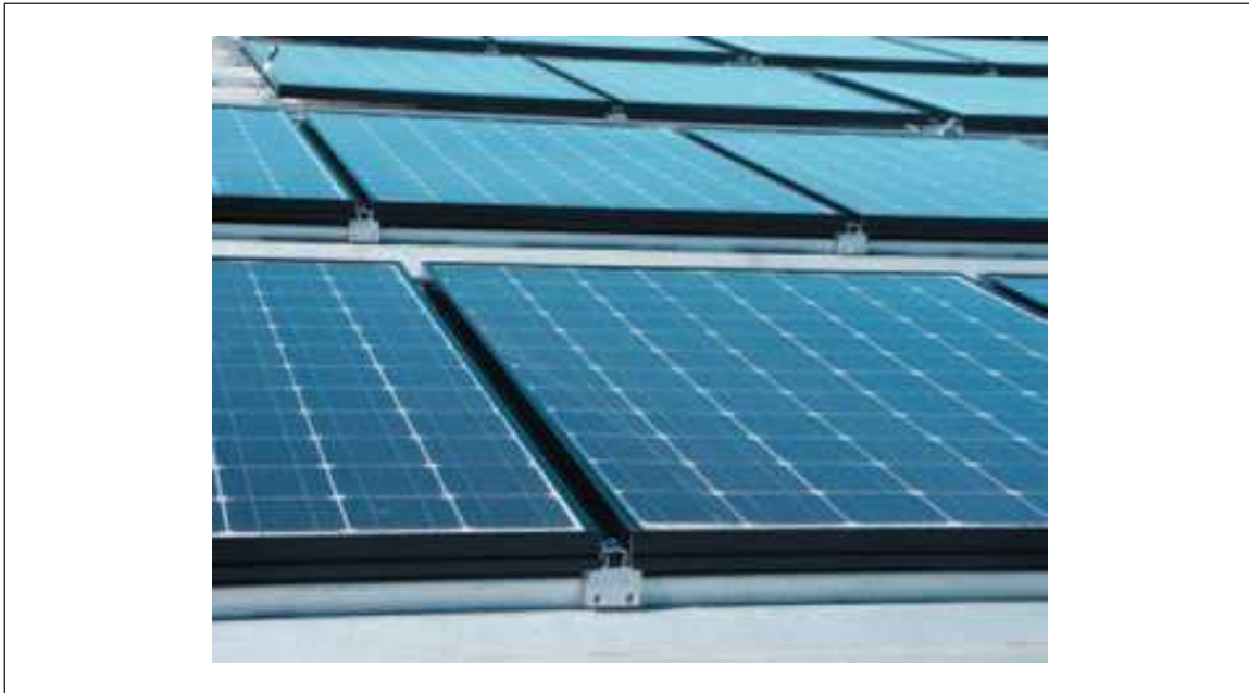
Fig. 10. Solar panels secured to standing seam roofs using external seam clamps
