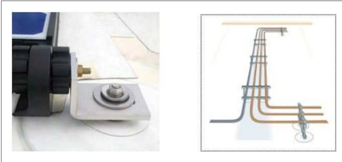
Figs. 2A and 2B. Examples of mechanical anchors used to secure equipment to the roof deck or roof framing
