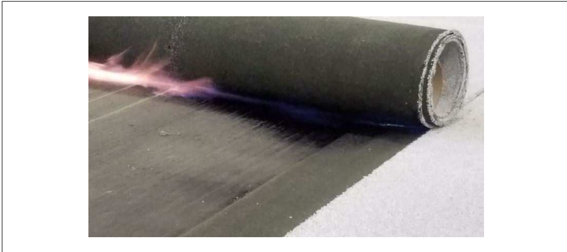
Fig. 1. Torch application of upper ply; note adhesive pooling at the leading edge of the roll
