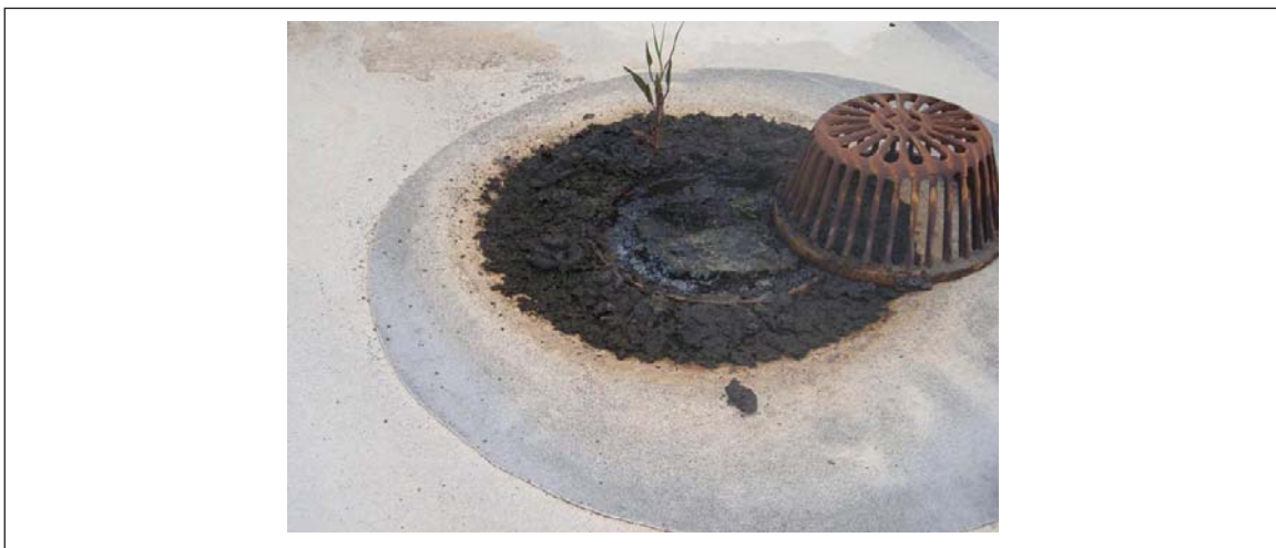
Fig. 3.1-2. Clogged roof drain
