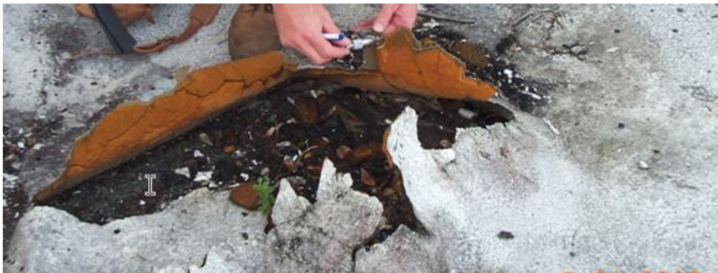
Fig. 3.1-11. Spray polyurethane foam flaking and delaminating
