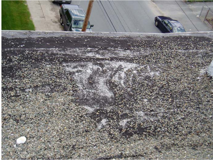
Fig. 3.1-10. Scrim showing where gravel is missing
