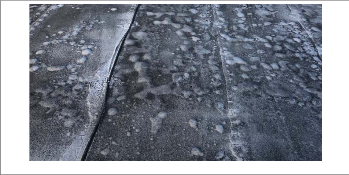
Fig. 3.1-8. Severe blistering of a built-up roof
