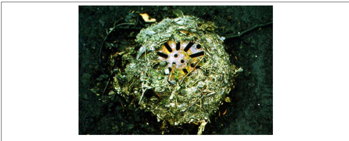
Fig. 3.1-1. Debris blocking roof drain
