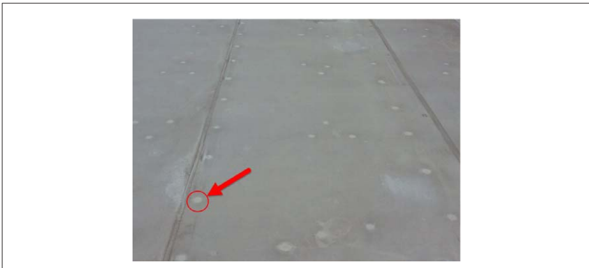
Fig. 3.1-5. Mechanically attached PVC cover with lighter areas over plastic stress plates that may indicate plasticizer loss and increase in brittleness
