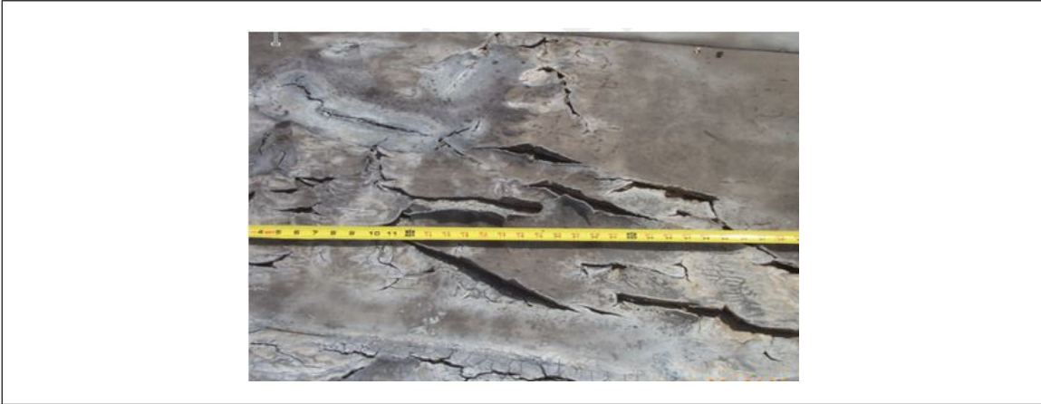
Fig. 3.1-6. Shrinkage and embrittlement of a thermoplastic single-ply roof with flaking of an incompatible asphaltic coating
