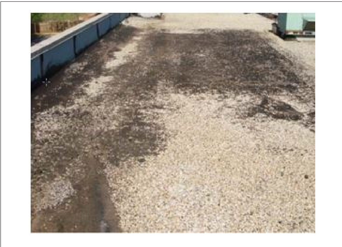
Fig. 3.1-9. Built-up roof with discolored area where water ponds (note exposed roof areas missing gravel)
