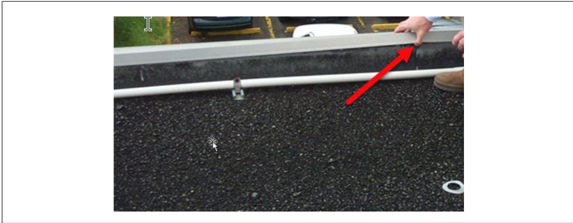
Fig. 3.1-3. Flashing easily lifted (follow appropriate safety procedures when near the roof edge)
