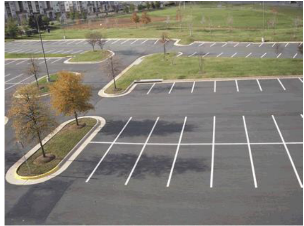
A Parking Lot with Curb-Opening Inlets
