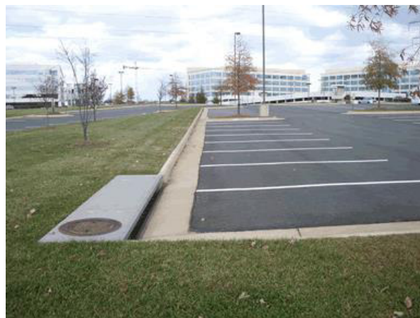
Concrete Curb/Gutter in a Parking Lot
