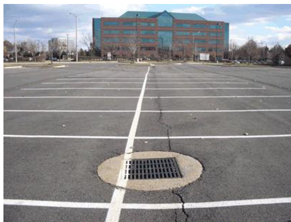
A Parking Lot with Grate Inlets
