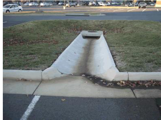
Connecting Two Drainage Systems
