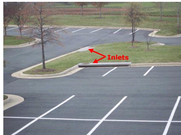
Two Curb-Opening Inlets at Low Spots
