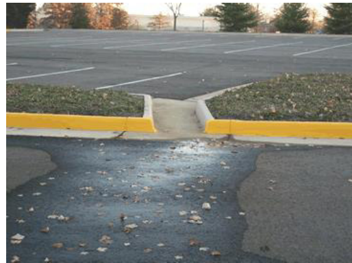
Splitting an Island for Water Passage
