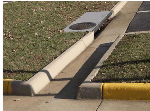
Terminating an Island next to a Curb
