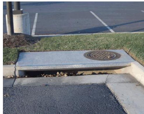
Figure 6 – A Curb-Opening Inlet
