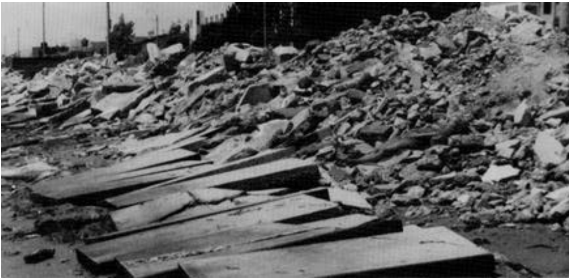
Figure B-42. concrete slab revetment, Alameda, CA
