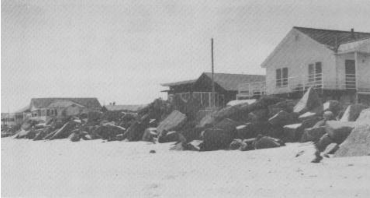
Figure C-7. Rubble-mound seawall, Fernandina Beach, FL
