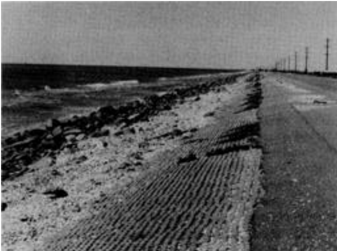
Figure 15. Gobi block revetment, Holly Beach, LA
