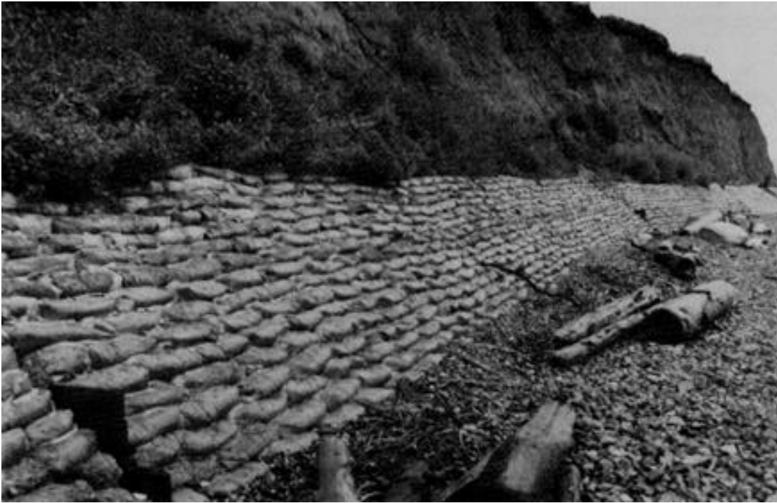
Figure B-34. Bag revetment at Oak Harbor, WA
