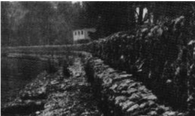
Figure D-28. Gabion bulkhead, possibly at Sand Point, MI
