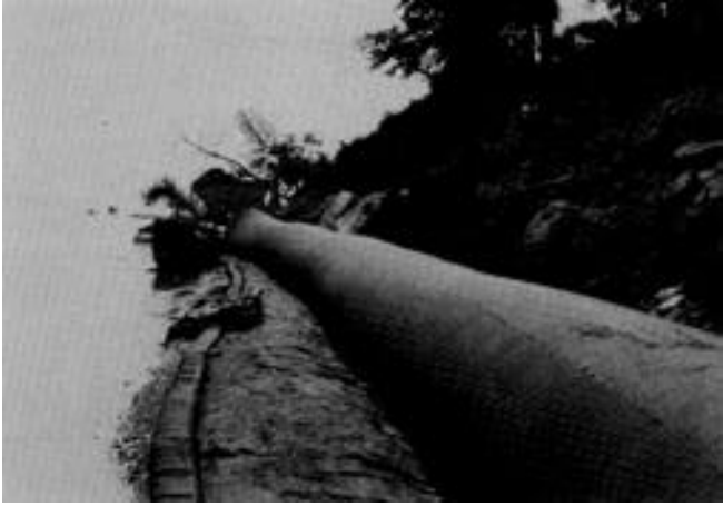
Figure D-25. Longard tube bulkhead, Ashland, WI
