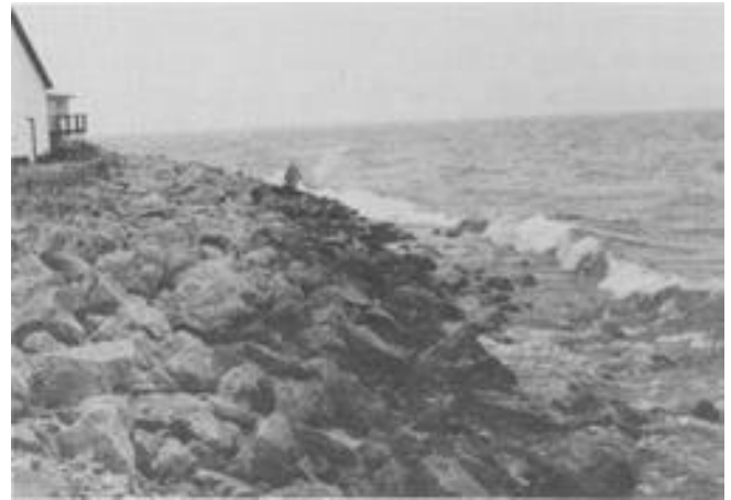
Figure B-1. Quarrystone revetment at Tawas Point, MI
