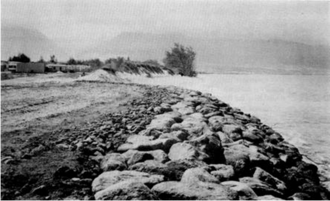
Figure B-5. Field stone revetment at Kekaha Beach, Kauai, HI
