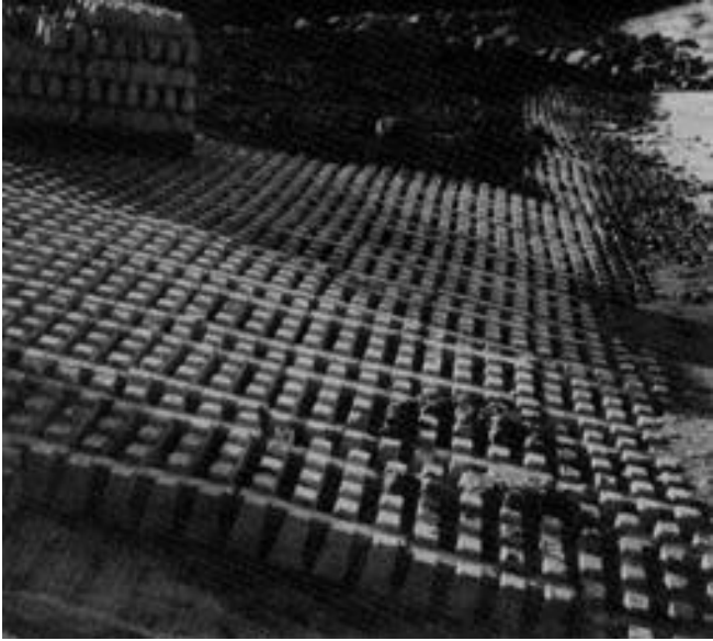
Figure B-17. Turfblock revetment, Port Wing, WI
