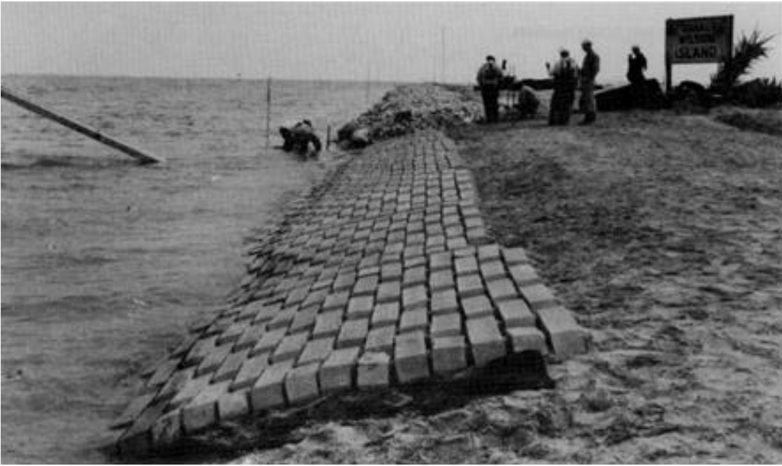
Figure B-30. Terrafix block revetment, Two Mile, FL
