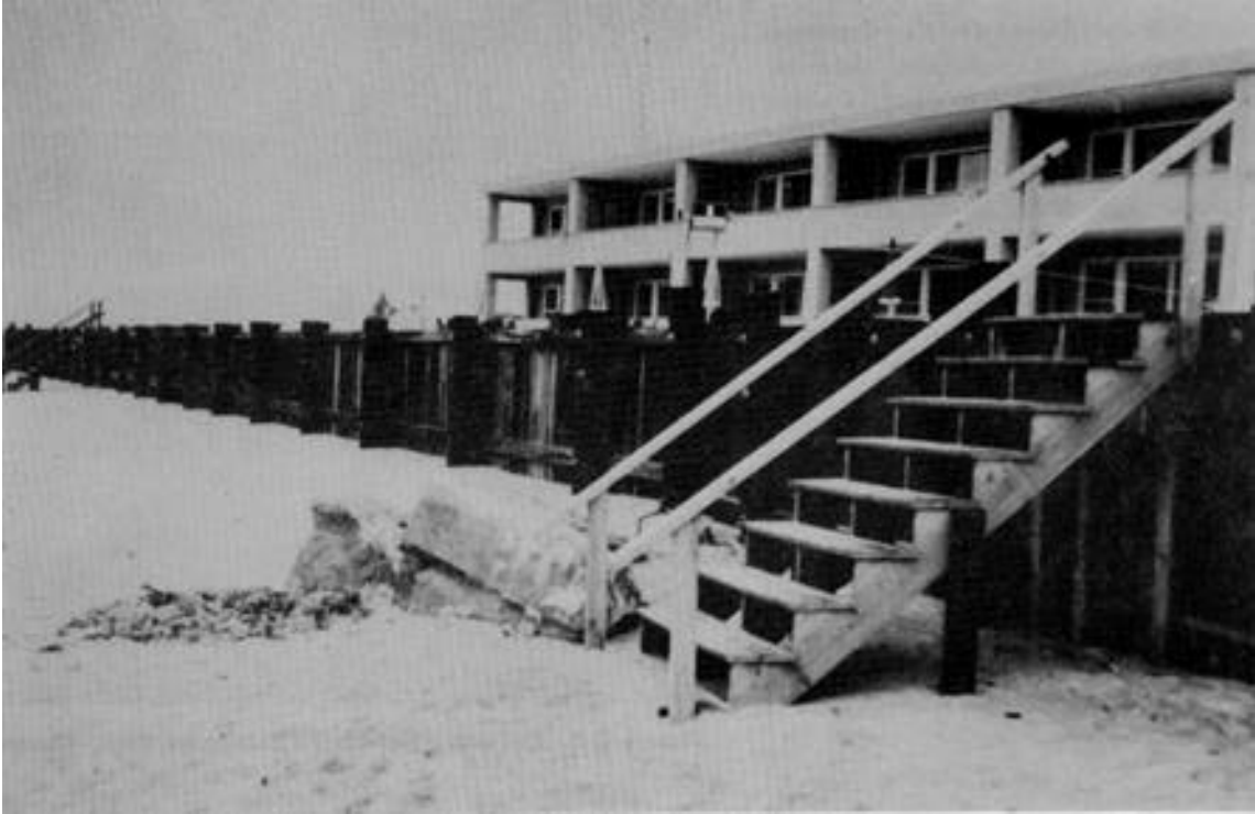
Figure D-3. Timber sheet-pile bulkhead, possibly at Fort Story, VA
