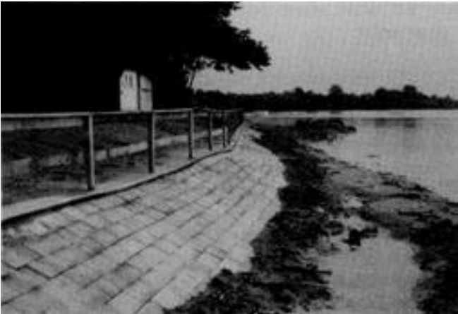
Figure B-26. Shiplap block revetment, Benedict, MD
