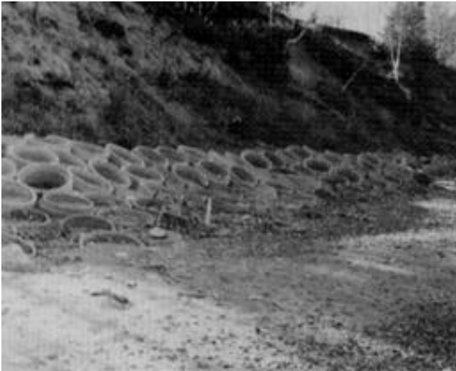
Figure B-19. Nami Ring revetment, Little Girls Point, MI
