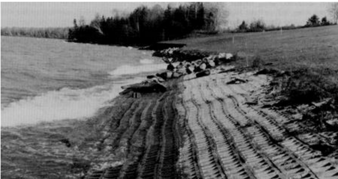
Figure B-24. Concrete control block revetment, Port Wing, WI
