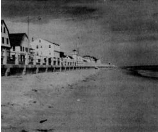
Figure D-8. Concrete slab and King-pile bulkhead
