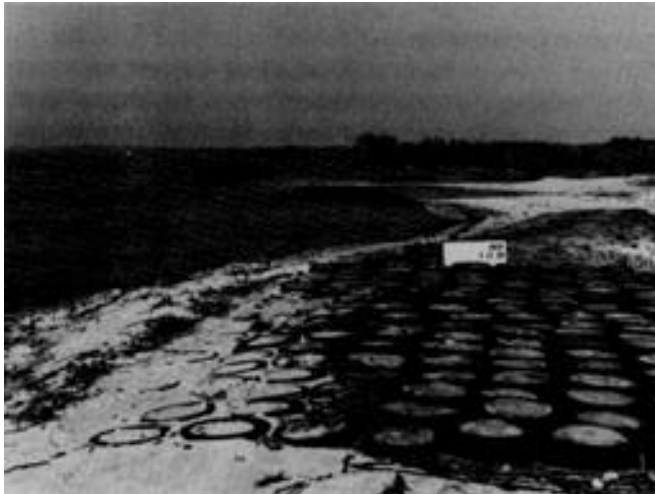
Figure B-46. Tire mattress revetment, Fontainebleau State Park, LA
