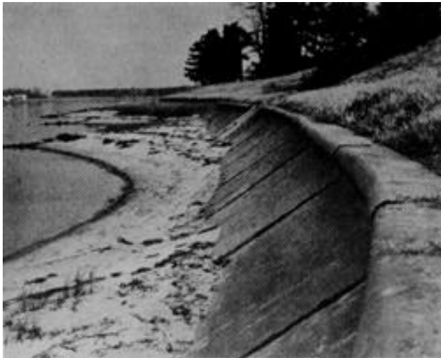
Figure B-12. Formed concrete revetment, Pioneer Point, MD
