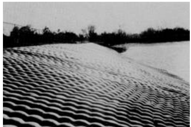
Figure B-32. Fabriform revetment, location unknown
