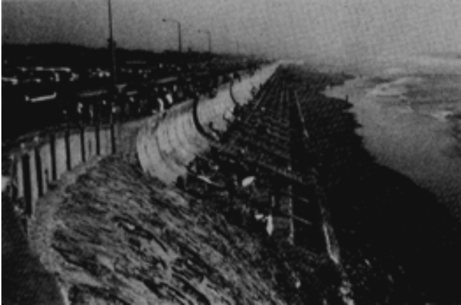
Figure C-5. Combination stepped- and curved-face seawall, San Francisco, CA
