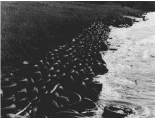
Figure D-21. Stacked rubber tire bulkhead, Port Wing, WI
