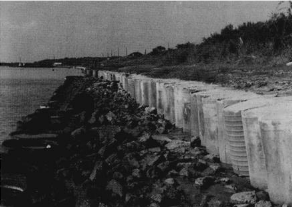
Figure D-23. Used concrete pipe bulkhead, Beach City, TX
