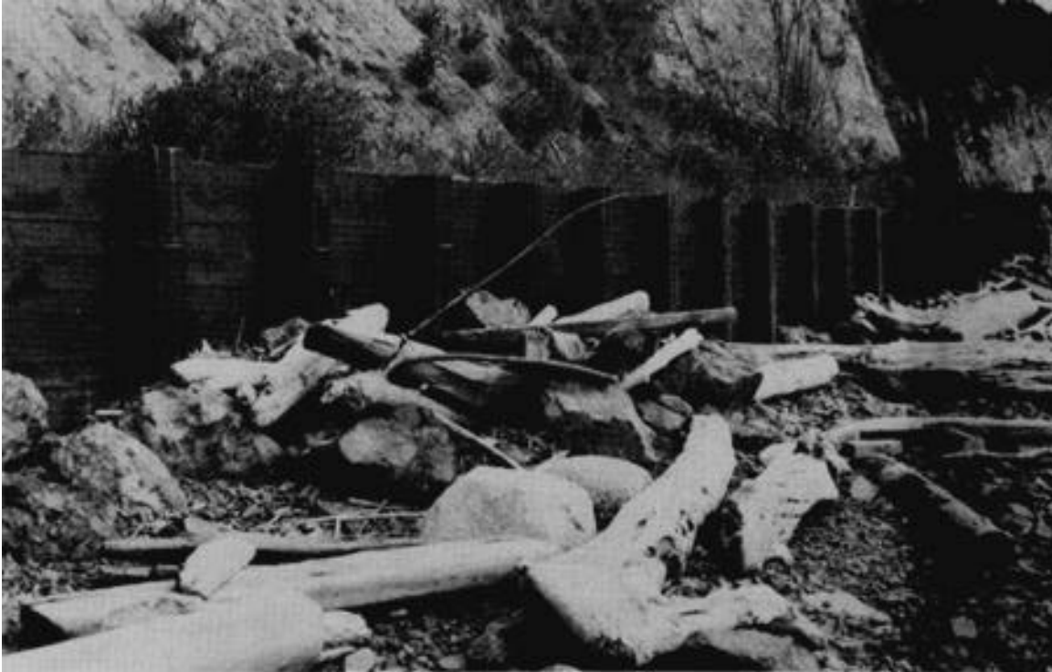
Figure D-12. Treated timber bulkhead, Oak Harbor WA
