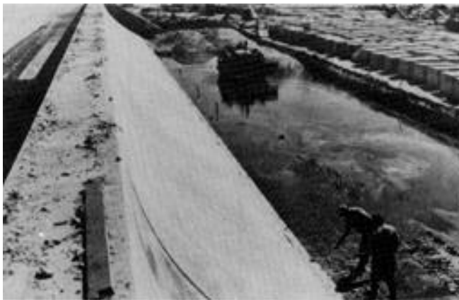
Figure C-1. Curved-face seawall, Galveston, TX
