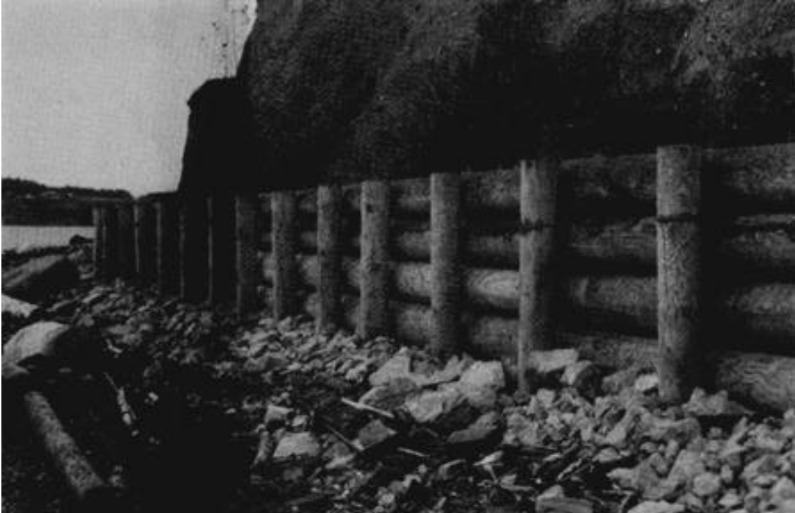
Figure D-14. Untreated log bulkhead, Oak Harbor, WA
