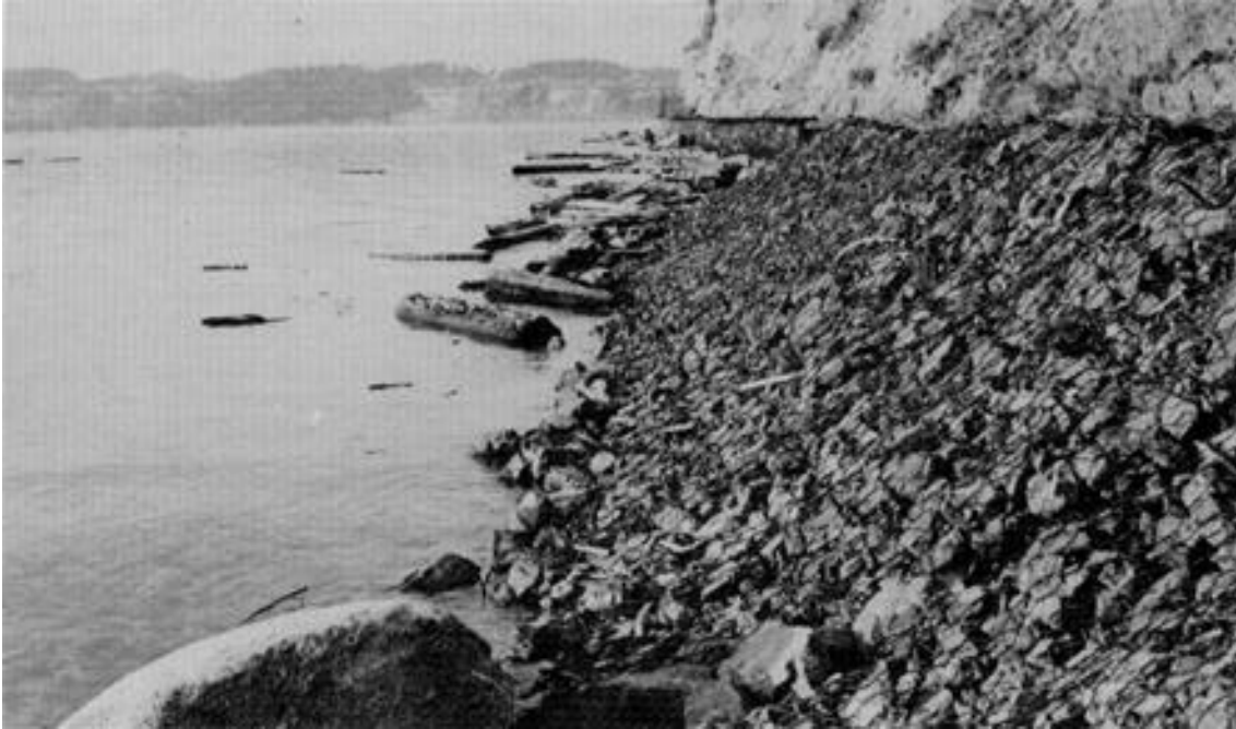
Figure B-36. Gabion revetment, Oak Harbor, WA
