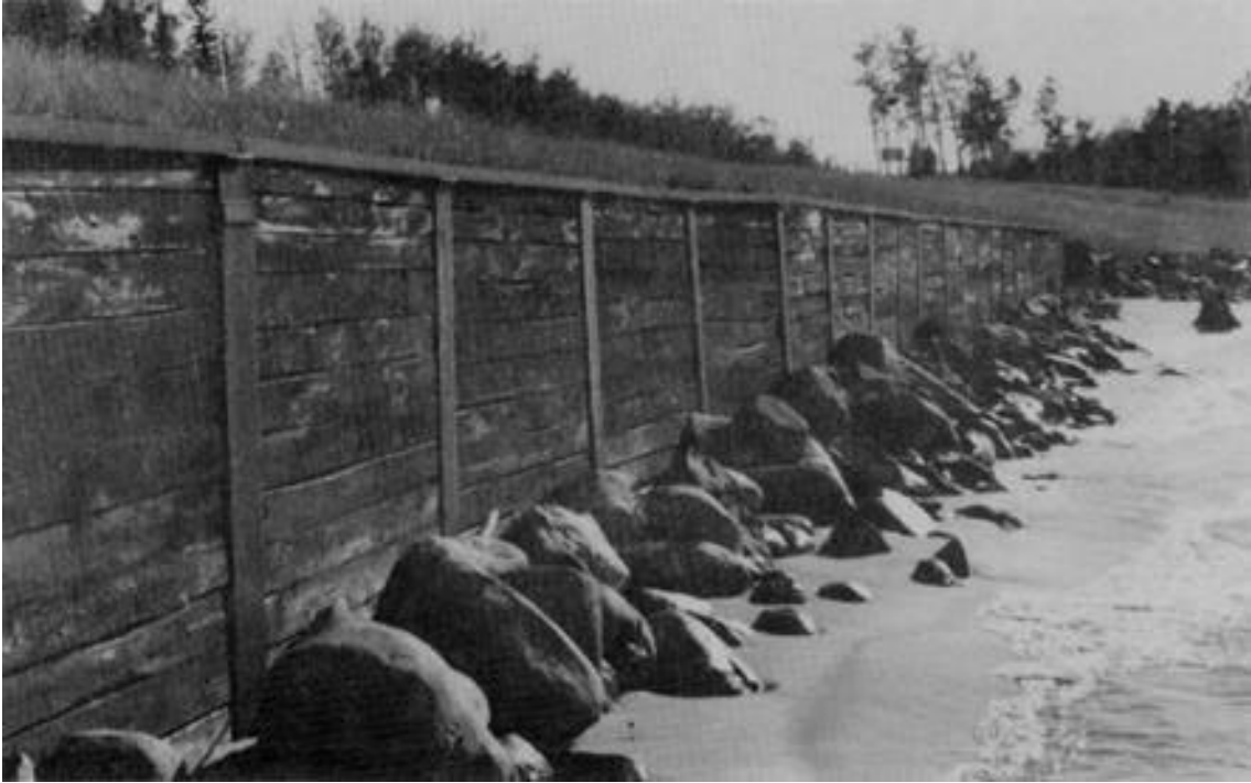
Figure D-10. Railroad ties and steel H-pile bulkhead, Port Wing, WI
