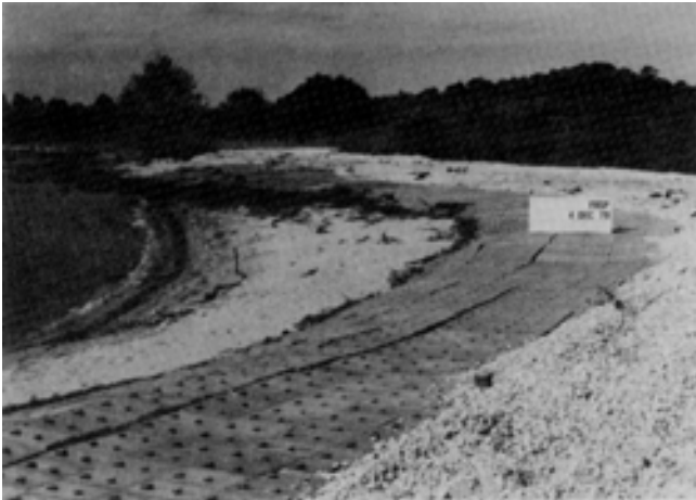
Figure B-21. Concrete construction block revetment, Fontainbleau, State Park, LA
