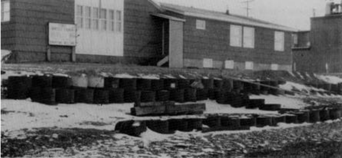
Figure B-38. Steel fuel barrel revetment, Kotzebue, AK
